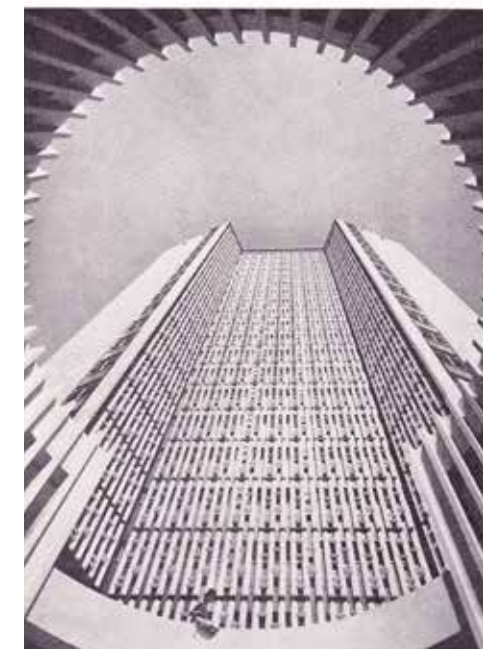
Livingstone House - tallest building in Salisbury - entire exterior by Terrastone Ltd
