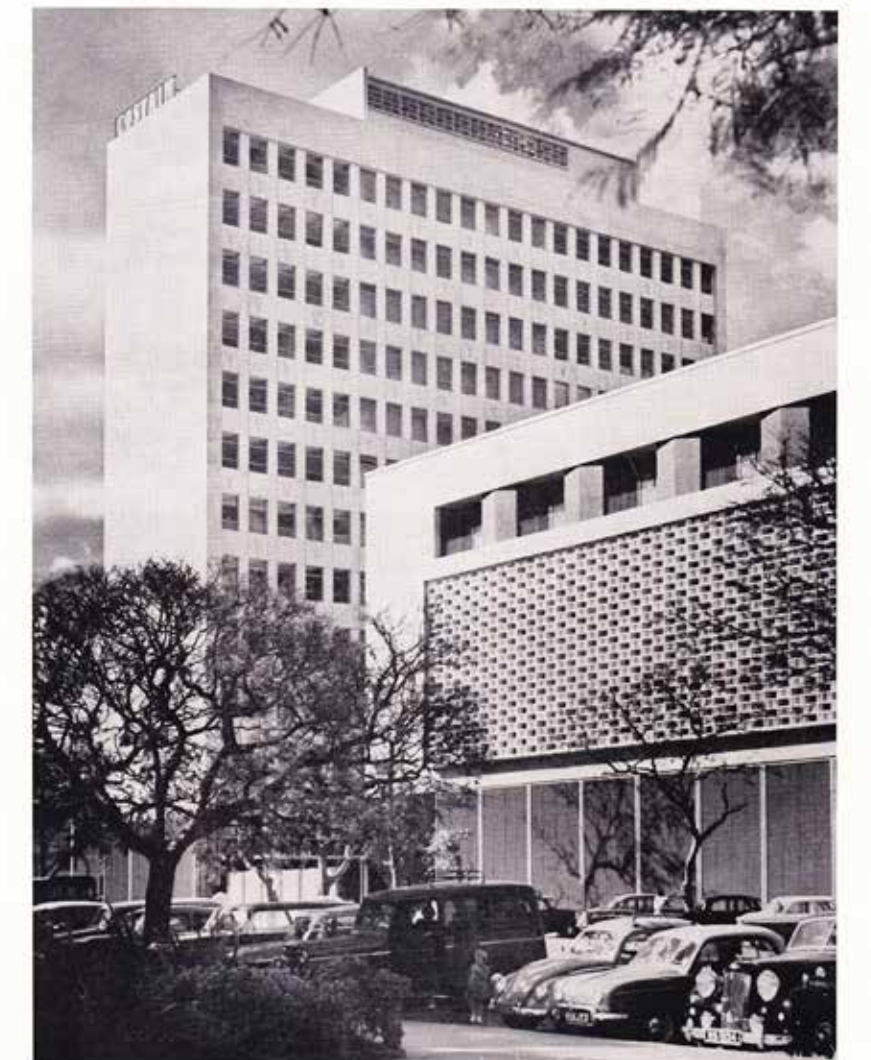
The delicate tracery of the brise soleil on the Salisbury Club and the clean sculpture of the reconstructed stone on the office block.
