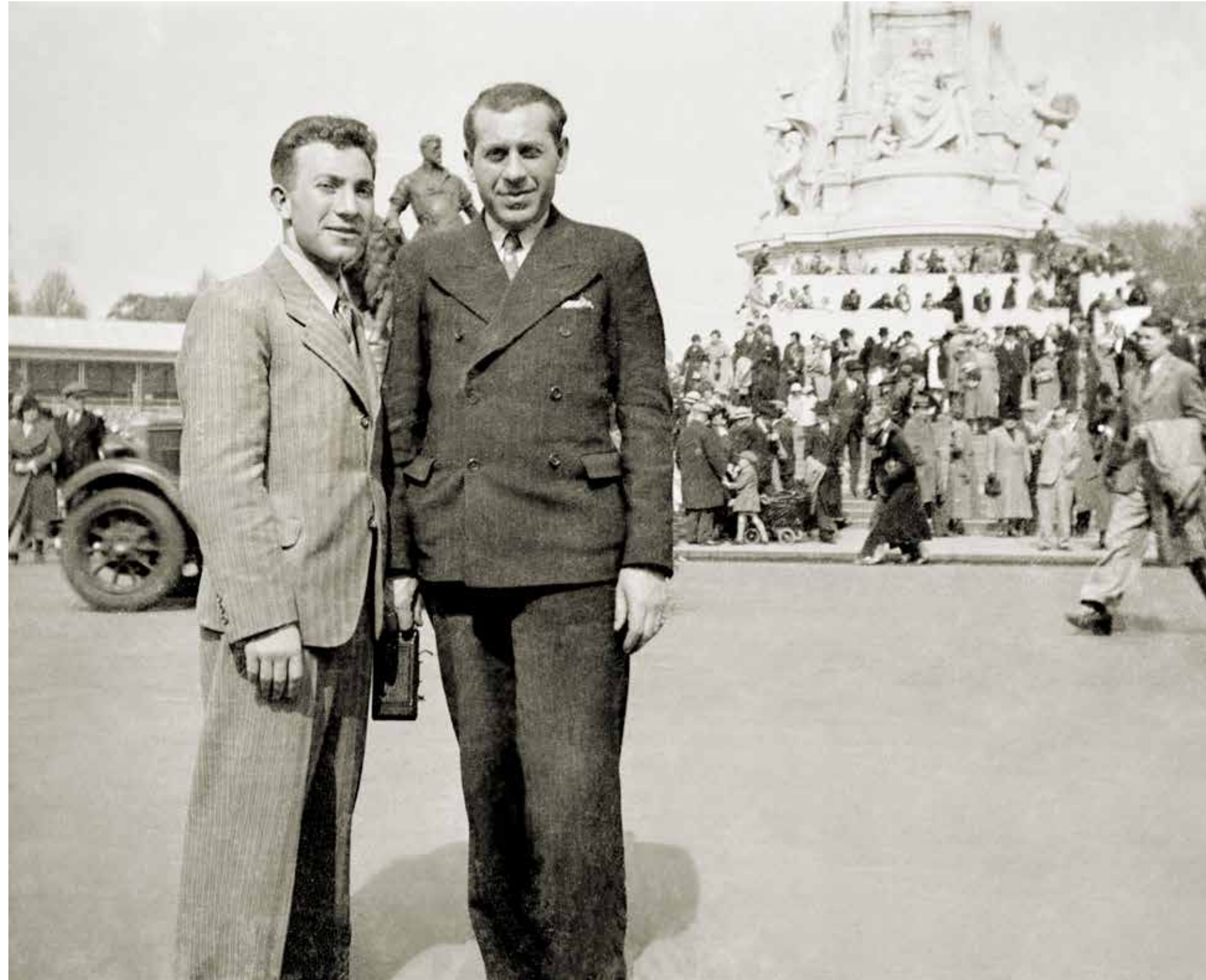
London, Buckingham Palace, King George V Silver Jubilee 1935. Photo dated according to scaffolding around the monument in the background which was uniquely surrounded by scaffolding for the press. David Chudy (left) and older brother Bernard.
