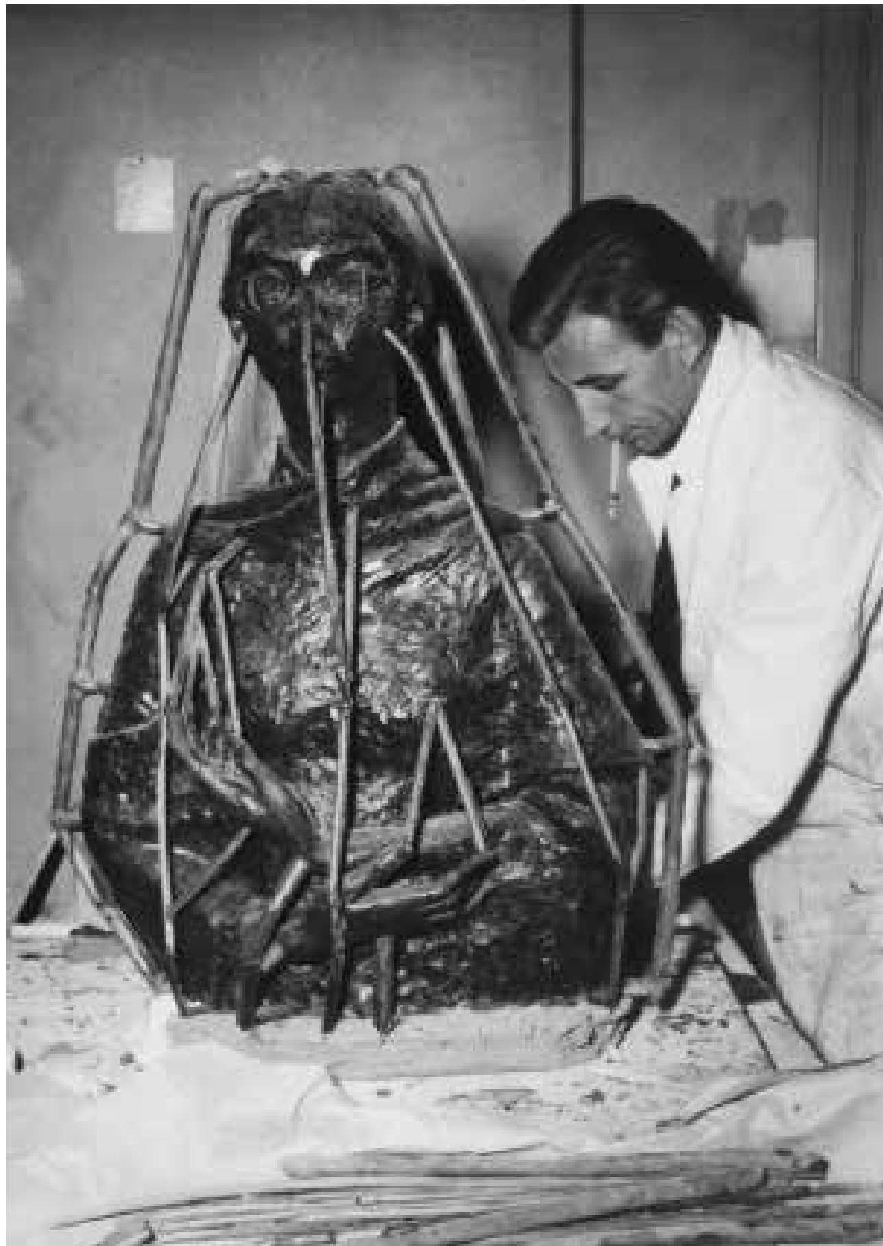
Wax channels are added to guide the molten bronze and avoid air gaps in the final cast
