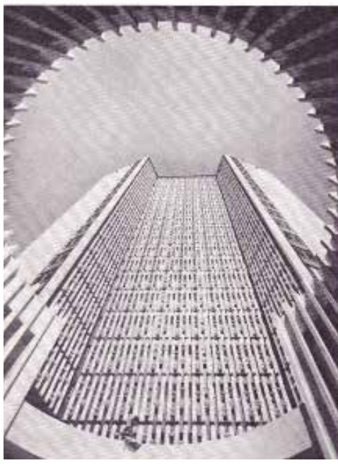
Livingstone House - tallest building in Salisbury - entire exterior by Terrastone Ltd
