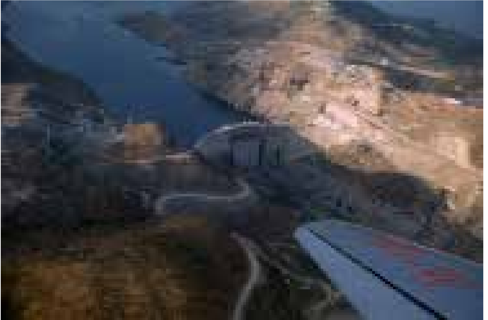
Aerial view of Kariba Dam construction (late 1950's), the world's largest dam by volume - circa 1956.
